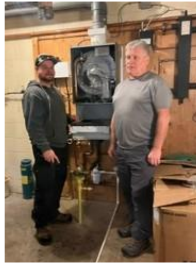
Dan McIntosh and NexGen employee inspecting the heat exchanger.
