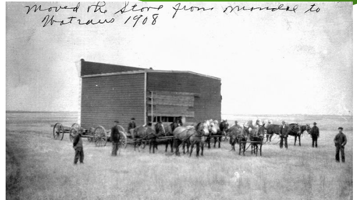
1908 Businesses moved their buildings from Mandel to Watrous when the CNR changed the rail line from Mandal to Watrous.
