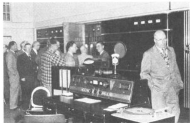
Visitors in the Transmitter Room — C.B.K.
